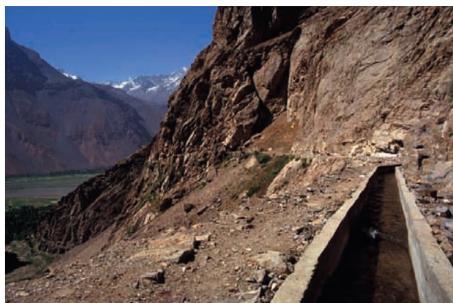
Picture 2.9: Water channel in Barrushan located in a rock face some 130m above the power plant. Water channels are highly prone to be damaged by natural hazards. (Photo: T. Hoeck, July 2003)
