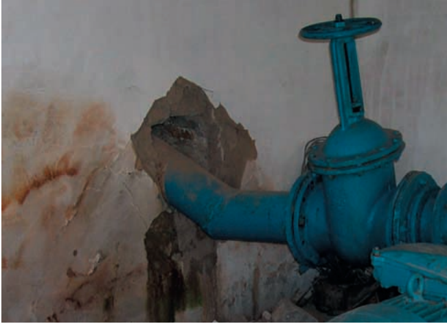
Picture 2.13: Melting snow and freezing water in combination with the engine vibration cause damage to the building and equipment. (Photo: T. Hoeck, June 2003)
