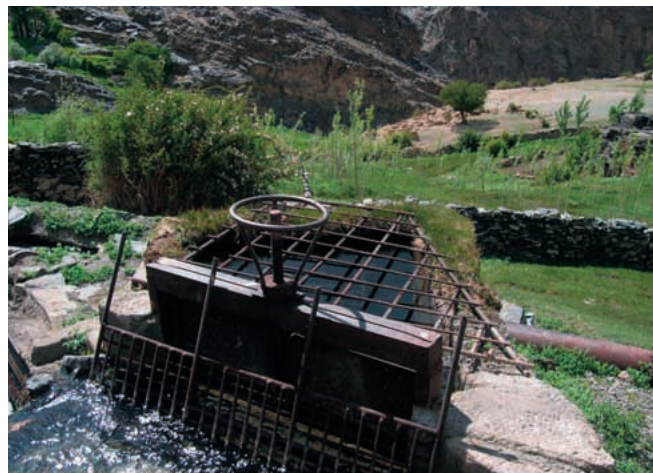
Picture 2.18: Water for the MHPS is diverted from the irrigation channel and stored in a very small forebay tank. Water supply is insufficient to operate the 80kW turbine at full capacity. (Photo: T. Hoeck, June 2003)
